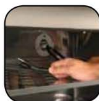
Throughwall Access Port
